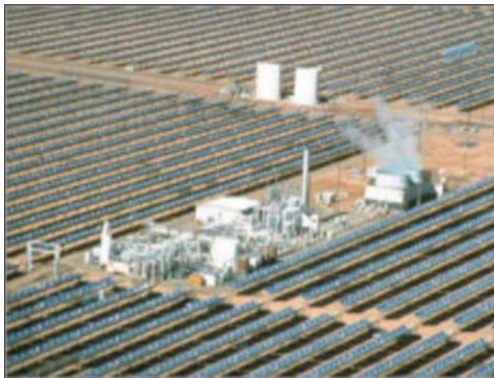
The Solar Electric Generating Station IV power plant in California has many parallel rows of parabolic trough collectors that track the sun. The cooling towers at right show water plumes rising into the air. White water tanks are in the background. Photo by Sandia National Laboratory
