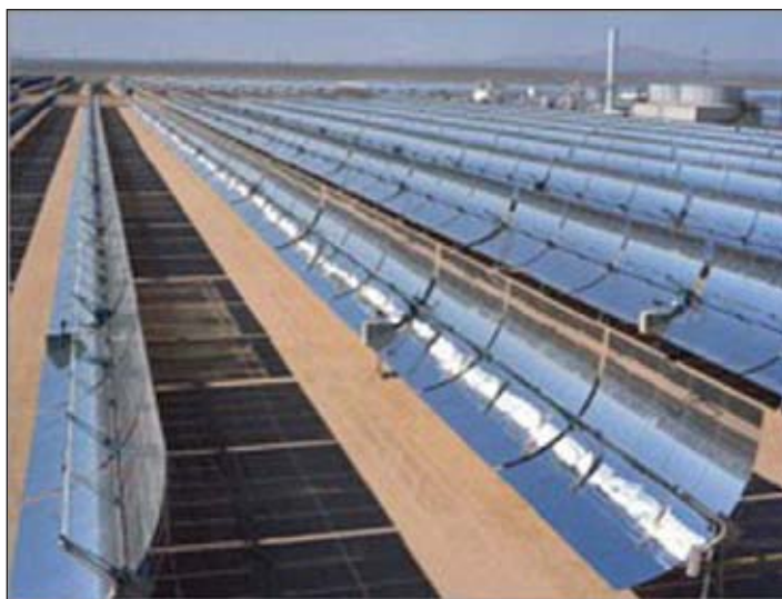
The Solar Electric Generating Station IV power plant in California has many parallel rows of parabolic trough collectors that track the sun. The cooling towers at right show water plumes rising into the air. White water tanks are in the background. Photo by Sandia National Laboratory
